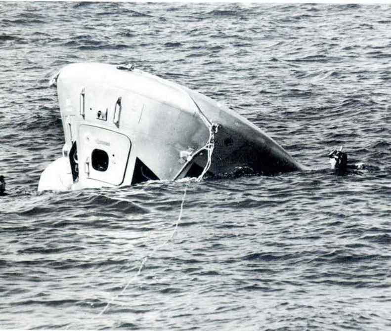
"Stable two," an engineering euphemism for upside-down, was one of the ways that the command module could float, and this was the way that Apollo 7 splashed down. The astronauts hung from their restraining belts for a few minutes until three righting bags were inflated to flip the spacecraft. The photo sequence above and at right, not the actual Apollo 7 landing, shows a training session, one of many constantly held to drill recovery teams and astronauts. Not used in this exercise was the flotation collar, normally fixed around the command module, that provided insurance against swamping from water taken aboard through the open hatch.
