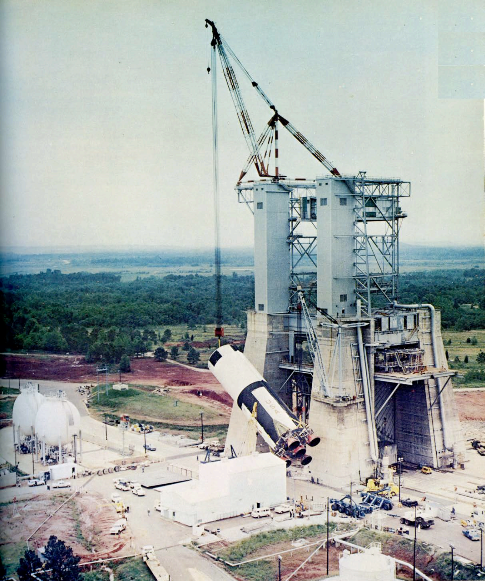
The first (S-IC) stage of the Saturn V launch vehicle being hoisted into the static test stand at Marshall Space Flight Center. This was the "battleship," or developmental test version of the stage, built heavily to permit repeated testing of flight-version working components. The first three flight S-IC stages were assembled at MSFC and tested in this stand. The massively reinforced construction of the 300-foot-tall stand was essential to withstand the 7.5 million pounds of thrust developed by the stage's engines during static testing.
