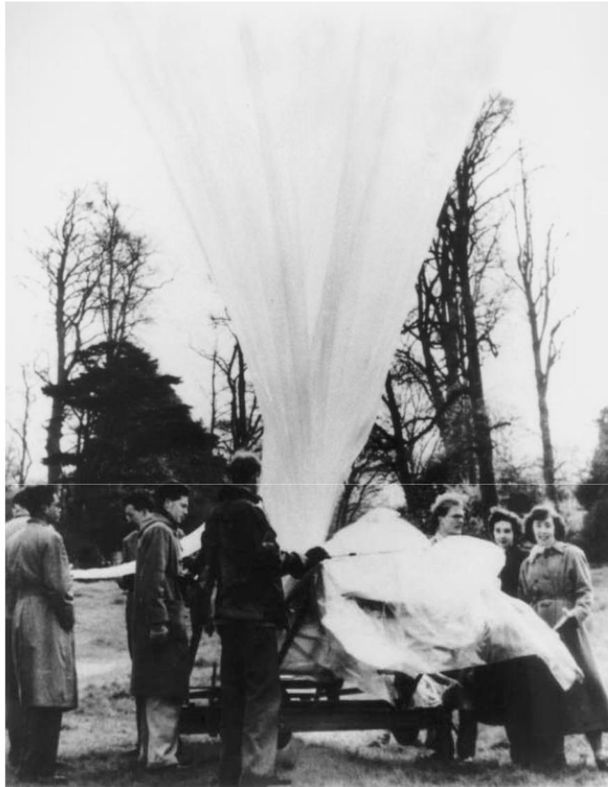
**Figure 1** A balloon ready for the ascent in the Sardinia area in July 1953. For the first time, emulsion stacks were made up of 40 stripped emulsions bound together between thick glass plates, wrapped and sealed and subsequently marked with X-rays.
